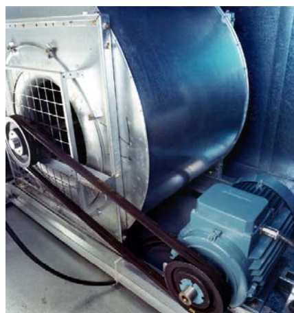
Figure 3 - Belt driven fan assembly
